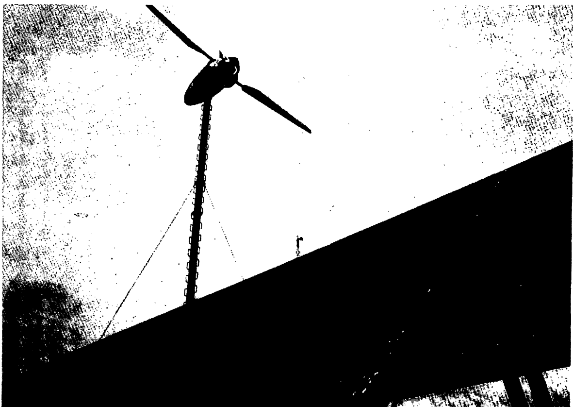
Figure 2 DWT 18kW wind generator (rotor dimension 9.5m) providing power for telephone exchange unit.
